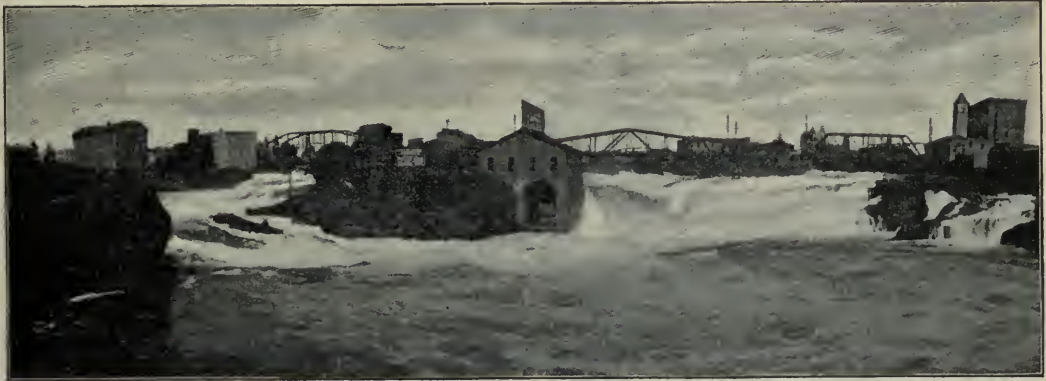
FIG. 310.—The falls in the Spokane River, around which the city of Spokane has grown.
